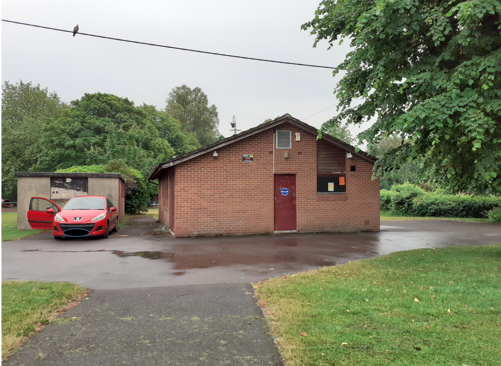
West elevation of the kiosk and storage building
