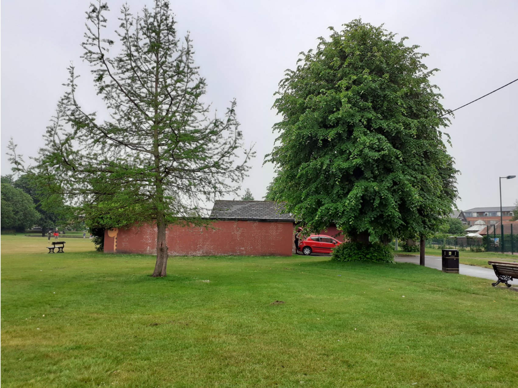
North elevation of storage building and kiosk
